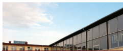
GYM HALL OF THE SCHOOL OF HIGHER VOCATIONAL EDUCATION IN NYSA – BUILDING O, OTMUCHOWSKA 68
